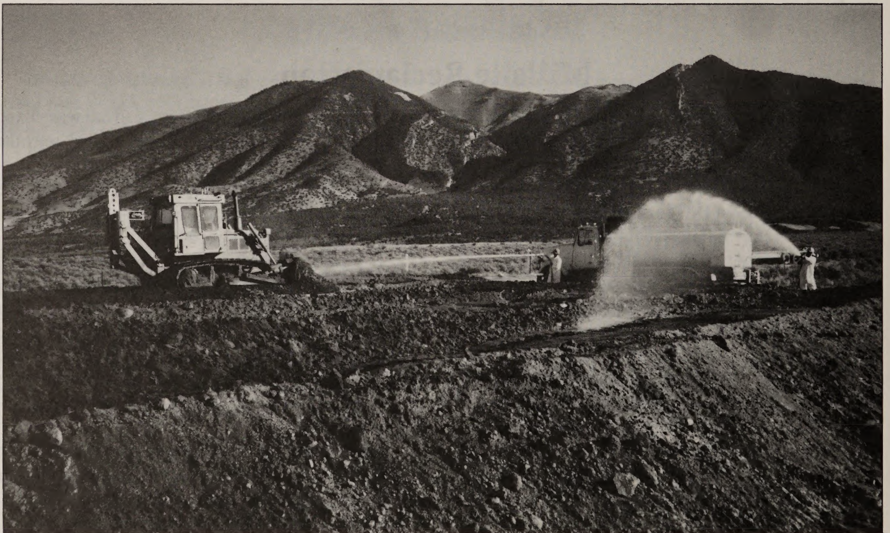
Figure 6. A dozer was used to mix the ore and reagents.
